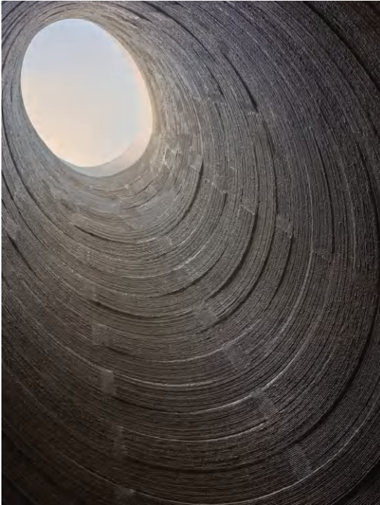
In addition to figurative and emotional reasons, the oculus also serves as a passive cooling system, directing warm air upward and expelling it outside. ©Jovian Lim
